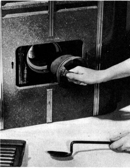
Removing plug-type door in pot-burner case. Off-set spoonlike implement in foreground is burner lighter. Small wad of paper or asbestos saturated with fuel oil is placed in lighter and lighted; then implement is inserted into burner until oil in burner is ignited by it.
